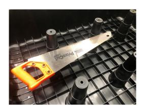
To reduce the CLEVA POD® down to the 150mm Step Down height, cut all the CLEVA POD® legs off at the 1st cone marking.
