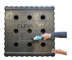
Cut the marked section out from the CLEVA POD®.
