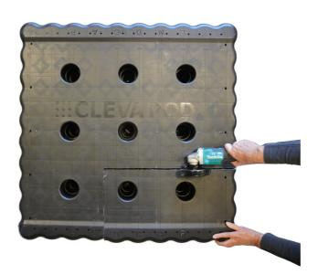
Cut the marked section out from the CLEVA POD®
