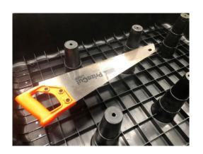
To reduce the CLEVA POD® down to the 150mm Step Down height, cut all the CLEVA POD® legs off at the 1st cone marking.
