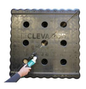
Cut the marked section out from the CLEVA POD®
