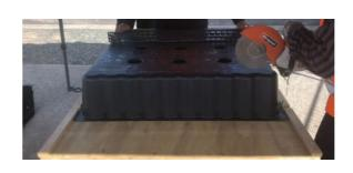
Before securing the guide rails with 32mm self-tapping wood screws, ensure the CLEVA POD® fits snuggly between the guide rails.
