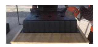
Before securing the guide rails with 32mm self-tapping wood screws, ensure the CLEVA POD® fits snuggly between the guide rails.
