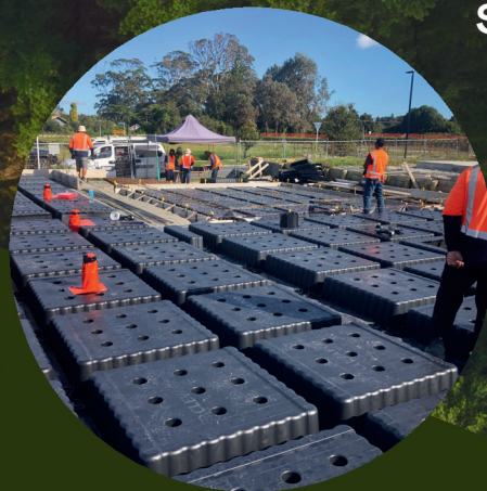
Clean work sites No polystyrene in sight!
